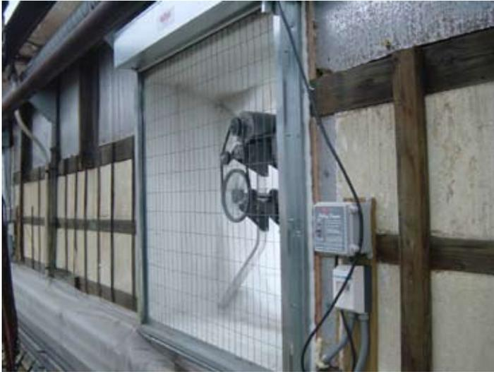
*Kube Pak Corp. in Allentown, N.J., installed rollup fan shutters (RollSeal, Inc., Bremen, AL) reducing air leakage and energy loss when the exhaust fans are turned off.*
