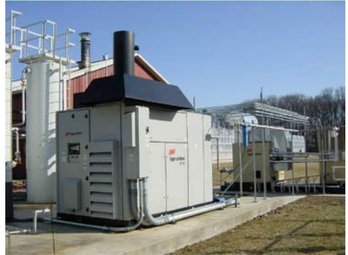
*An example using alternative energy (cogeneration) is this landfill gas-fired microturbine system installed at the Rutgers EcoComplex greenhouse in Bordentown, N.J. (Ingersoll Rand Co., Portsmouth, NH).*
