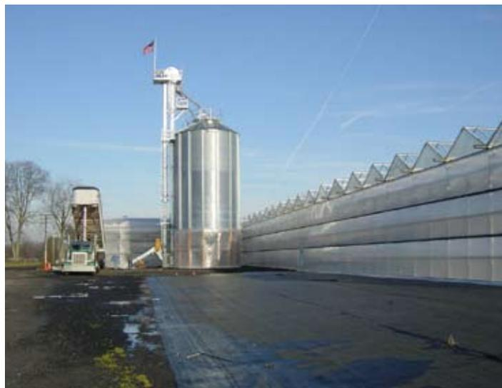
*Plainview Growers in Allamuchy, N.J., installed an alternative energy system delivering wood pellets to a newly installed biomass boiler. The plan is for the biomass boiler (Crone, B.V., Netherlands) to be fired in the near future with biomass pellets produced on the farm (from switchgrass and/or Miscanthus).*
