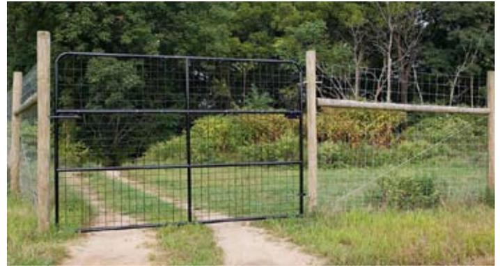
*A properly installed “H-braced” corner and gate.*
