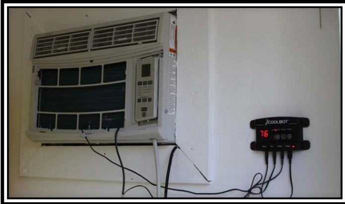
The CoolBot unit overrides the thermostat of a household window AC unit, keeping it running until reaching the temperature selected – much below the limits of the AC's own thermostat.
