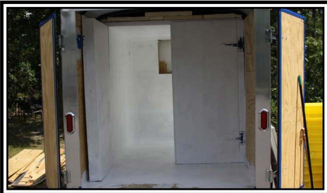
Inner doors were built to partition the cooler from the storage area
