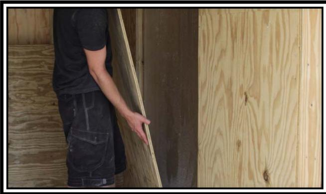
Framing covered two-thirds of the walls, front, and ceiling to create the cooler box.
