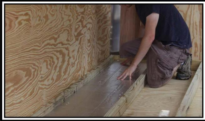
A standard 2 x 4 frame was built of pressure treated lumber to cover the entire floor.
