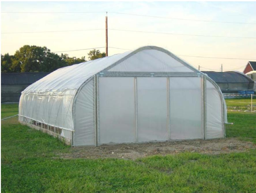
**Photo 2. Finished high tunnel with manual roll-up sides.**
