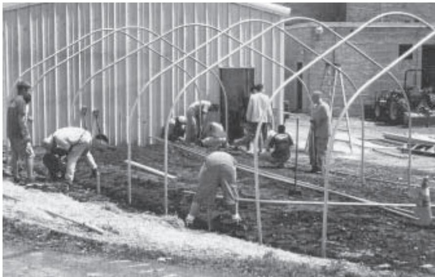
**Fig. 1. Vocational agricultural students at North Potter High School, Ulysses, Pa., assisting Penn State extension specialists and county extension personnel in the construction of a 17 × 36-ft (5.2 × 11.0-m) high tunnel located at the high school.**
