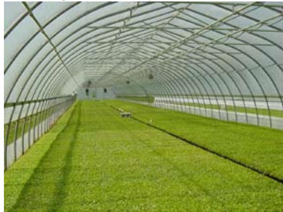
*Figure 1. Single span, naturally ventilated greenhouse covered with air-inflated double-layer polyethylene film. The crop is supported a few inches above the dirt floor. Photo: A.J. Both.*
