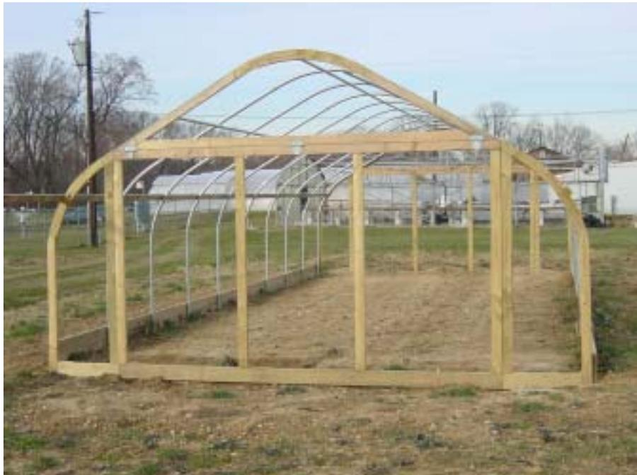
Fig. 1. High tunnel under construction showing a completely framed end wall.
